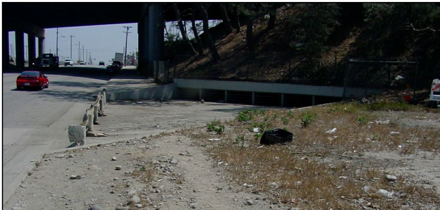
Figure 2-11 Inlet of Box Culvert on San Fernando Road under Interstate 5
