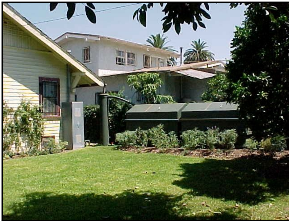
Figure 3-20 Fenceline Cistern at the Hall House
