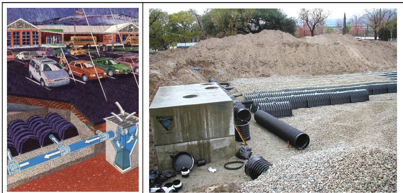
Figure 3-15 Subsurface Infiltration Devices
